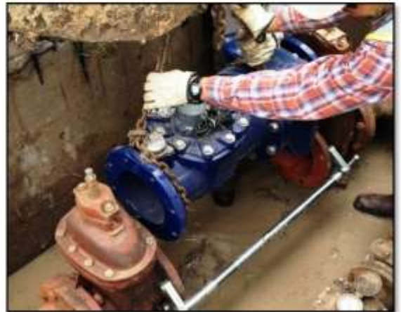
New Meter Installed
